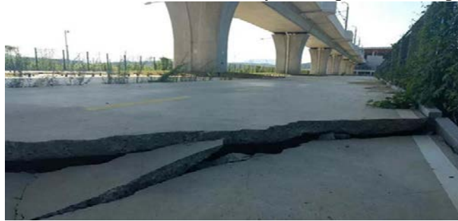
Figure 1 Subgrade and pavement of settlement section in road and Bridge Engineering
